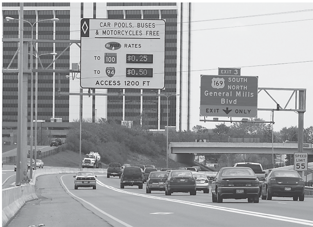
FIGURE 1 I-394 MnPASS high-occupancy toll lane.
