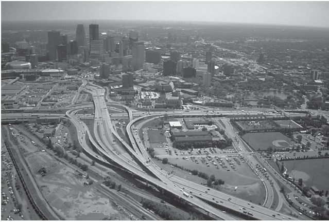
FIGURE 3 I-394 MnPASS lane entering downtown Minneapolis and I-94.
